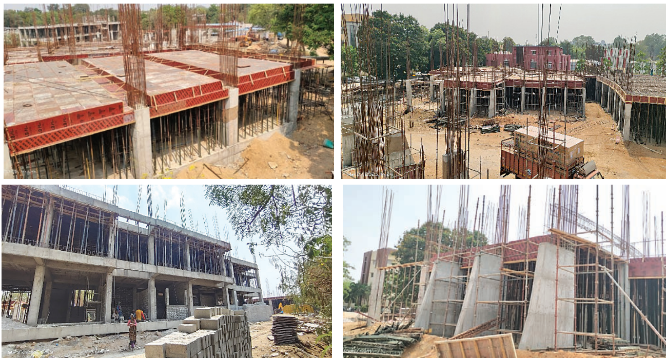
Fig. 6.16. Construction of Global Centre of Excellence on Millets building at ICAR-IIMR, Hyderabad
