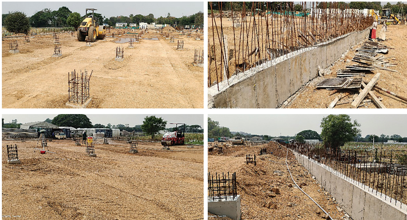
Fig. 6.17. Construction of Field Research Facility at ICAR-IIMR, Hyderabad
