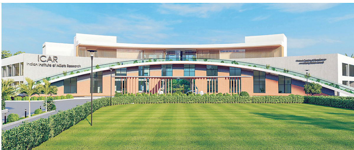
Upcoming Global Centre of Excellence on Millets building
