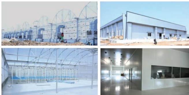
Fig. 9.19: Construction of Field Research Facility at ICAR-IIMR, Hyderabad
