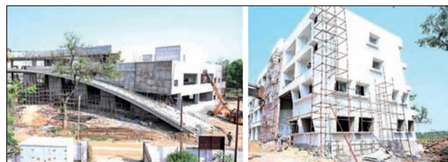
Fig. 9.18 Progress in Global Centre of Excellence on Millets building at ICAR-IIMR, Hyderabad
