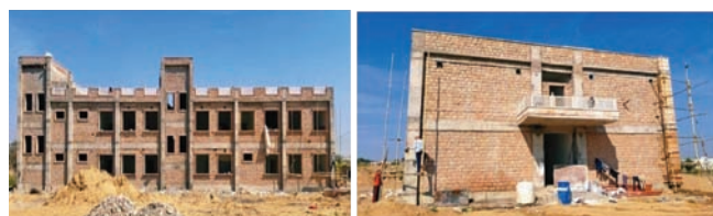
Fig. 9.20 Infrastructure development at Regional Research Station at Barmer
