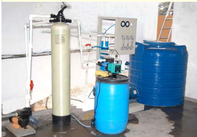
New RO based water purifying plant at NRCS
